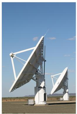
The IF system currently has a 256MHz instantaneous bandwidth, and RF is transmitted over optical fiber to the initial (Fringe Finder) correlator. It (and all other
