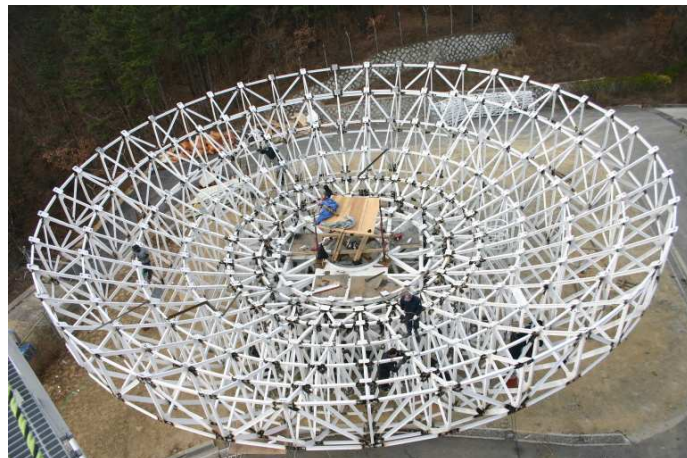
Figure 3: KVN antenna back structure at Ulsan site
