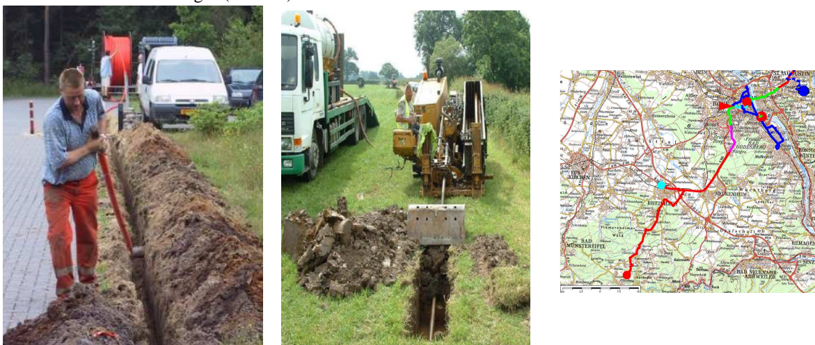
Figure 4: Last-mile fibre works at Westerbork (left), Jodrell Bank (center), and future line to Effelsberg (right).
