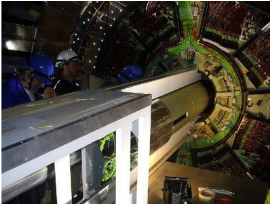
Figure 8: Insertion of the barrel pixel. Foreground: installation cassette with temporary rails. Background: patch panel PP0 with the insertion hole. The detector is just sliding in. The green part with the slit is the supply tube with the hole for the beam pipe suspension.
