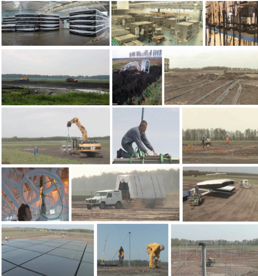
Figure 4: Some of the stages involved in building LOFAR – producing and storing the antenna hardware, preparing the fields, placing the cabinets, digging in the cables and finally deploying the HBA and LBA antennas.
