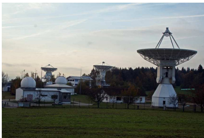
Figure 3: The new sky line of the Geodetic Observatory Wettzell: in the background are the new TWIN telescopes
