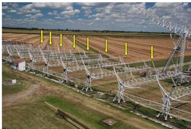
Fig. 1: Four receivers on 8 different cylindrical concentrators.
