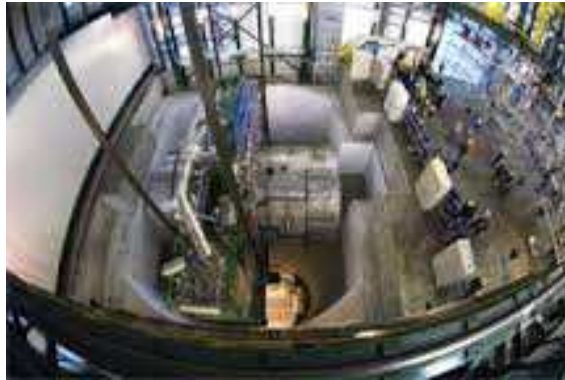
Figure 3: A snapshot of the historical lowering of YB0 into the experimental cavern.
