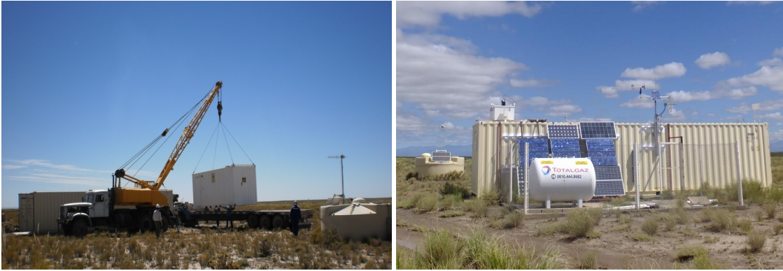
Figure 2: (Left) Replacing the old CLF container. (Right) The CLF after the upgrade was completed.
