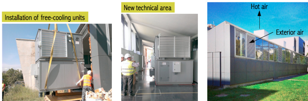
Figure 4: Free-cooling units being installed in PIC, in mid June 2014.
