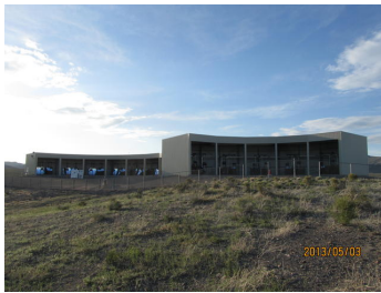
Figure 2: The lower building on the left is the main TA building contains 14 telescopes viewing 3-31° elevation. The taller building on the right has 10 TALE telescopes viewing 31-59° elevation above the main TA telescopes.
