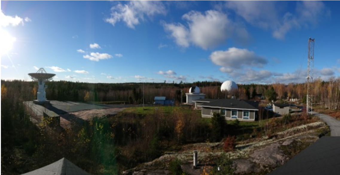
Figure 1: Overview of the Metsähovi Geodetic Research Station. The new VGOS radio telescope is on the left side, the main building with all the computer facilities (middle), the small radome behind the main building belongs to the SLR, and finally the big radome is part of the Aalto Metsähovi Radio Observatory. Photo: Markku Poutanen
