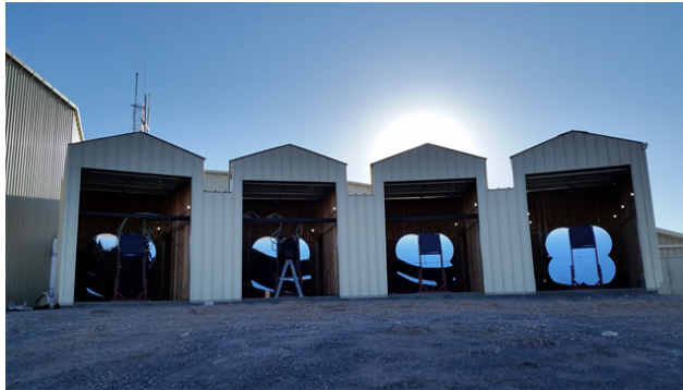
Figure 3: Picture of assembled 4 telescopes in the FD station at the north site of the TAX4 experiment.
