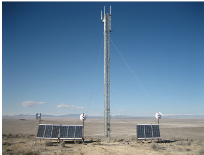
Figure 8: One of the constructed tower (SNCT).
