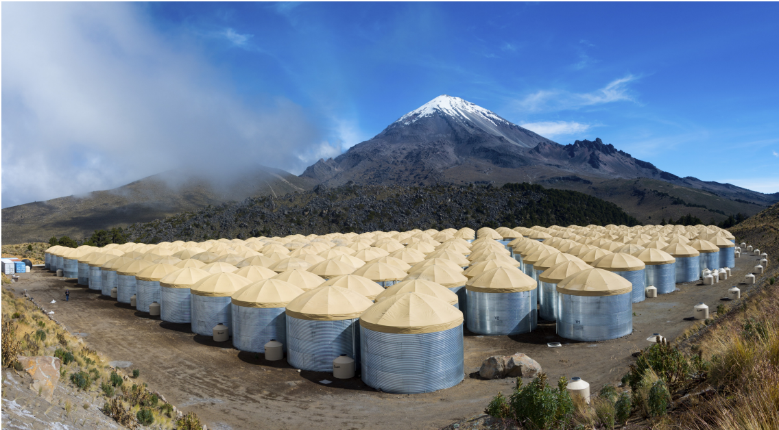
Figure 1: The HAWC site during the deployment of the outrigger array. The central dense tank array is shown with a space array of much smaller outrigger tanks around the perimeter of the platform.
