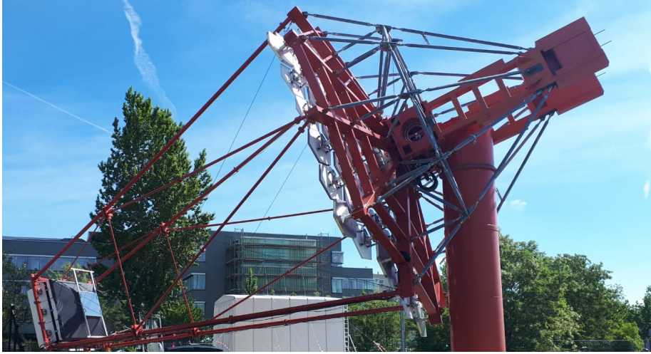
Figure 1: The NectarCAM camera in the MST structure at Berlin-Adlershof.
