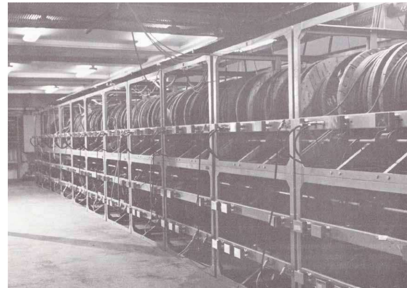
Figure 1: The correction for the direction dependent time delay for each element telescope was done by a series of switchable cable lengths per telescope, stored in the basement of the WSRT control building. Each telescope had a set of cables, totalling 1500 m in total, and switchable increments of 10 m (around 30 ns), at the intermediate frequency of 30 MHz) (E. Raimond, 1974)
