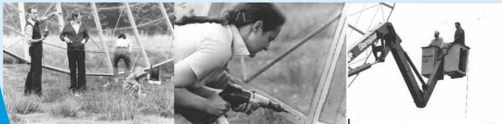
The pictures tell the story! We see (left) Ron Harten and family, (middle) Susan Simkin as hard working volunteer drilling screws at ground level, and (right) high up, Cees Slotje and Hans van Someren Greve. In one incident, a basket was accidentally driven into the reflector, but the antenna performance loss turned out to be minimal (and there were no injuries to our volunteers).
