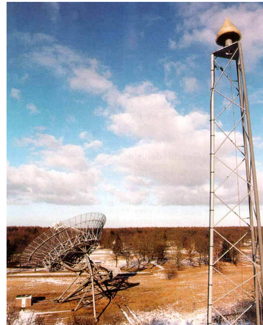
Figure 1. GPS Antenna mast at Westerbork in 1997.
