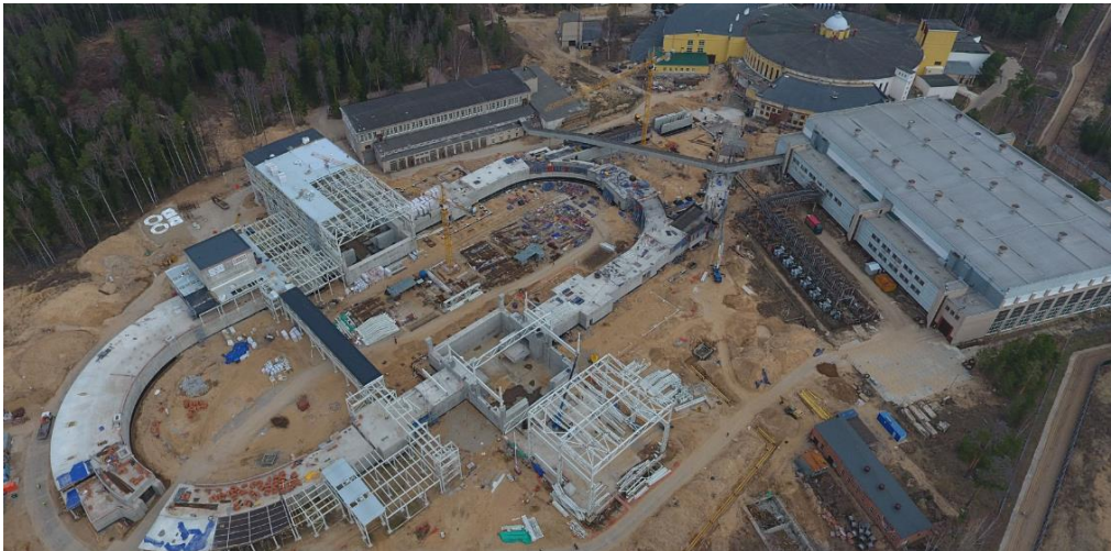
Figure 6: The construction site of the NICA collider.
