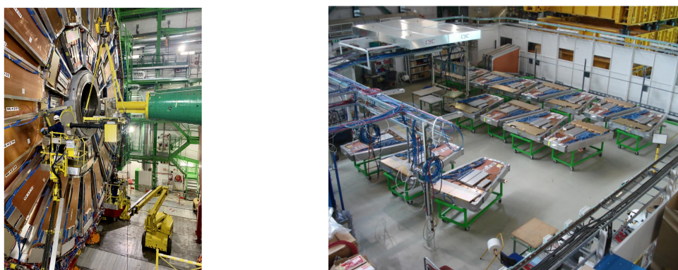
Figure 4: Left: Chamber extraction and reinstallation in the CMS underground cavern. Right: Refurbishment of the on-chamber electronics at SX5.
