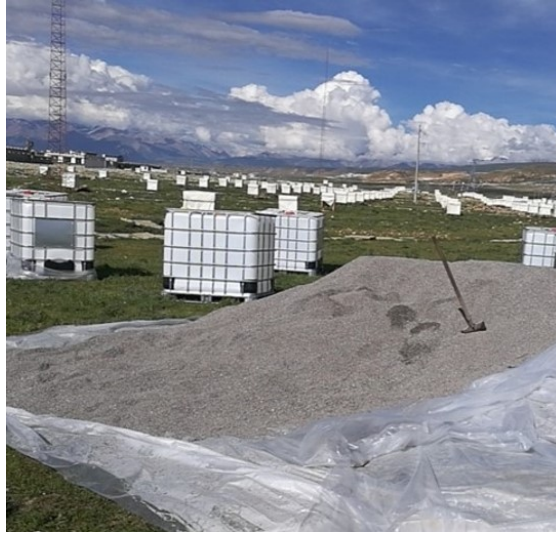
Figure 5: Sand cube(white tank in the front of picture) under construction
