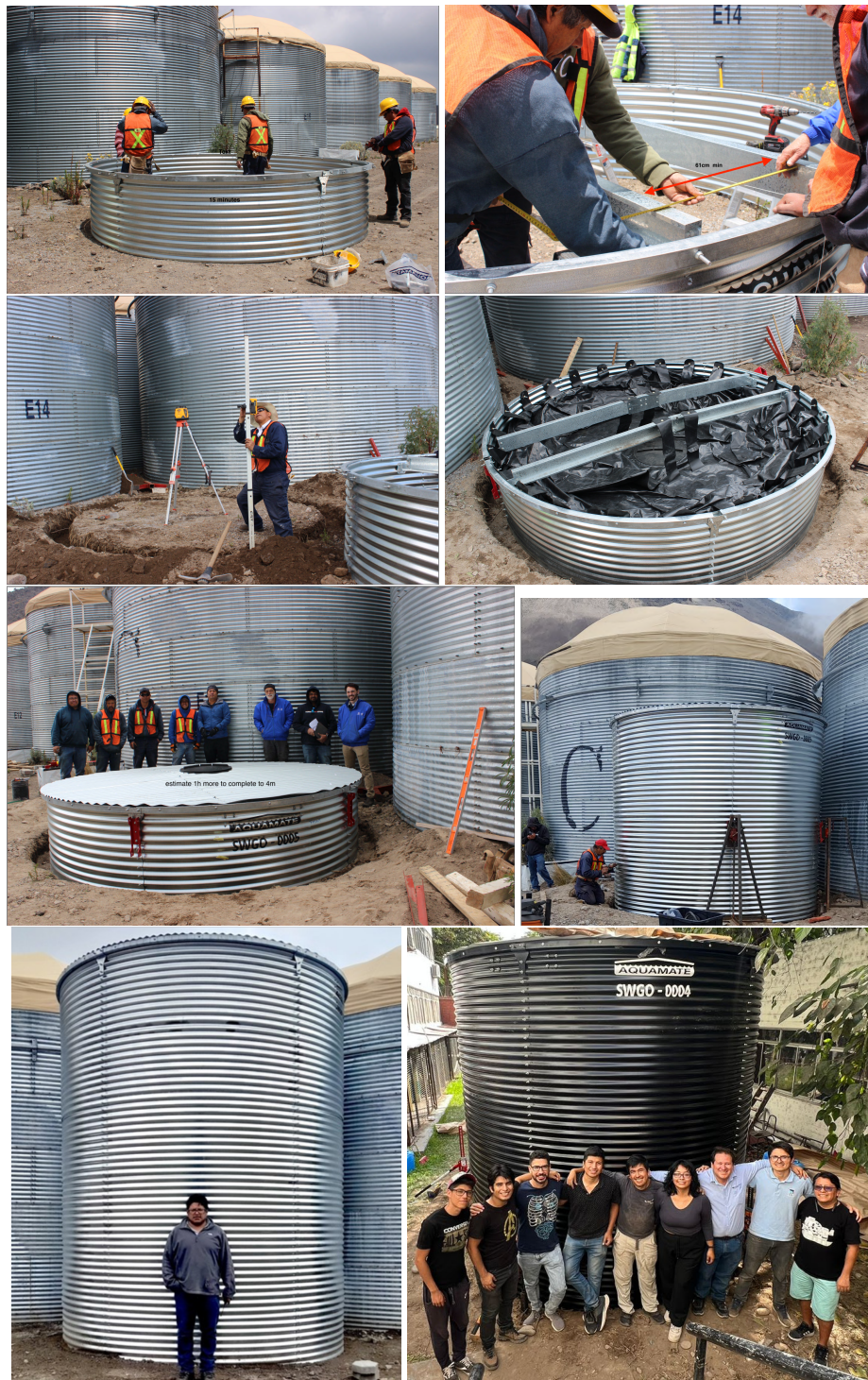
Figure 6: Steps followed to assemble the SWGO kit in HAWC and in Peru. a) bolt the top ring of the wall and the roof support bars, b) dig a trench and move the top ring in place, c) place the bladder inside the tank and bolt bladder support straps, d) bolt the roof panels and install the roof hatch and e) use the jacks to lift the tank and bolt lower rings. The photos in the bottom shows two different fully assembled SWGO kits at HAWC (4.3m height) and in Peru (3.6m height), both tanks have the same diameter of 3.6m.
