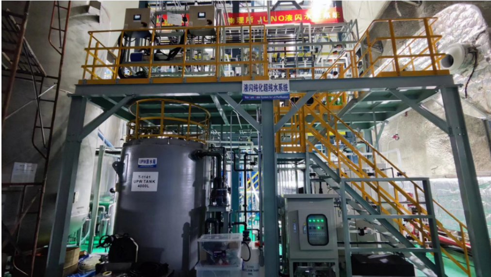
Figure 11: Ultra pure water plant
