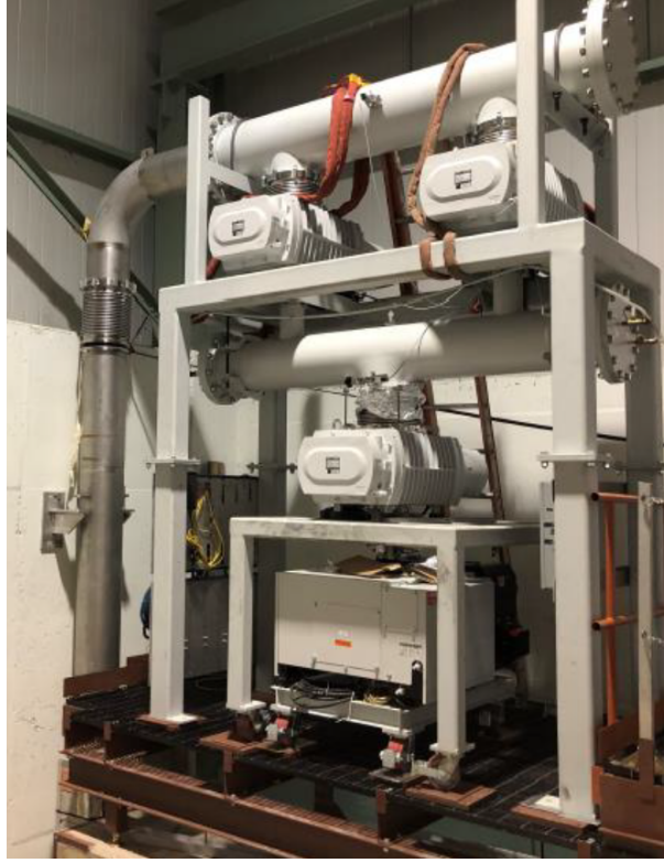
Figure 3: The pumping stack consists of three roots blowers and one backing pump. The 12" inlet piping goes down to the target cave and connects to the refrigerator through a gate valve
