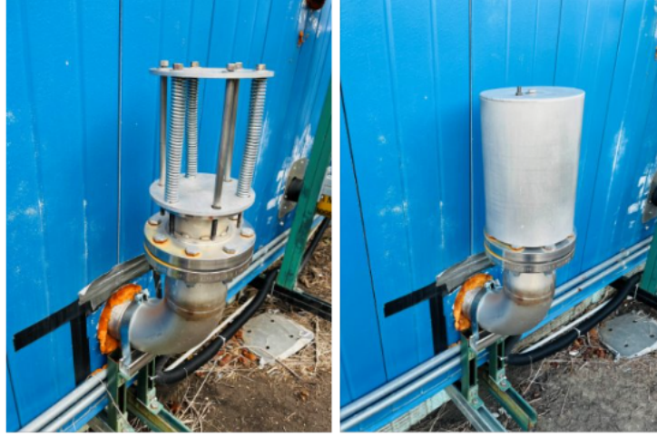
Figure 7: The operational relief valve of the magnet, the parallel plate valve is located at the outside of the experimental hall
