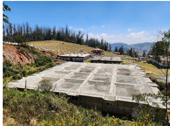
Figure 2: Photographs of the Akeno Muon Telescope (left) and the GRAPES-3 Muon Telescope in Ooty, India (right). Both use layered proportional counters with similar angular resolution.
