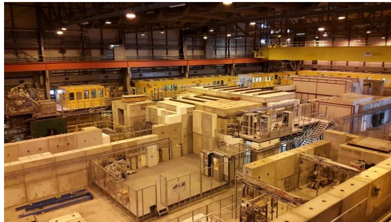
Figure 1 View from outside of the new GIF++ facility. The irradiation bunker as well as the preparation area and the electronic and service areas are visible. The total length of the facility is about 30 meters
